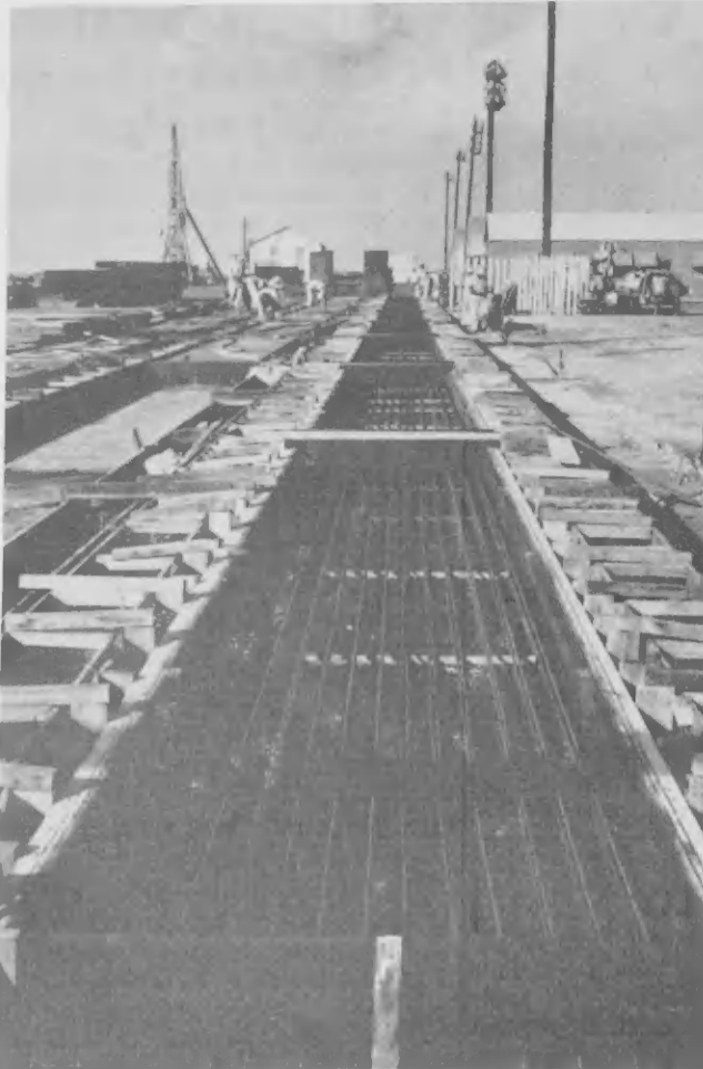
A CRANE lifts a seven-ton prestressed concrete slab from one of three stress beds in the lower yard storage area after the slab has cured in the form for three days. Steel tendons that give the slabs prestressed qualities, left, are elongated 18.7 inches more than their normal 300-foot lengths by a force of 18,600 pounds applied by stressing jacks.
